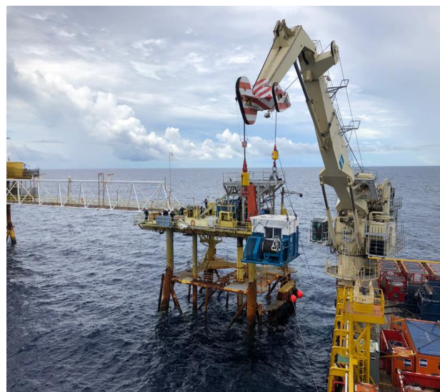
Plug & Abandonment Operation in the Nido AW-Platform
